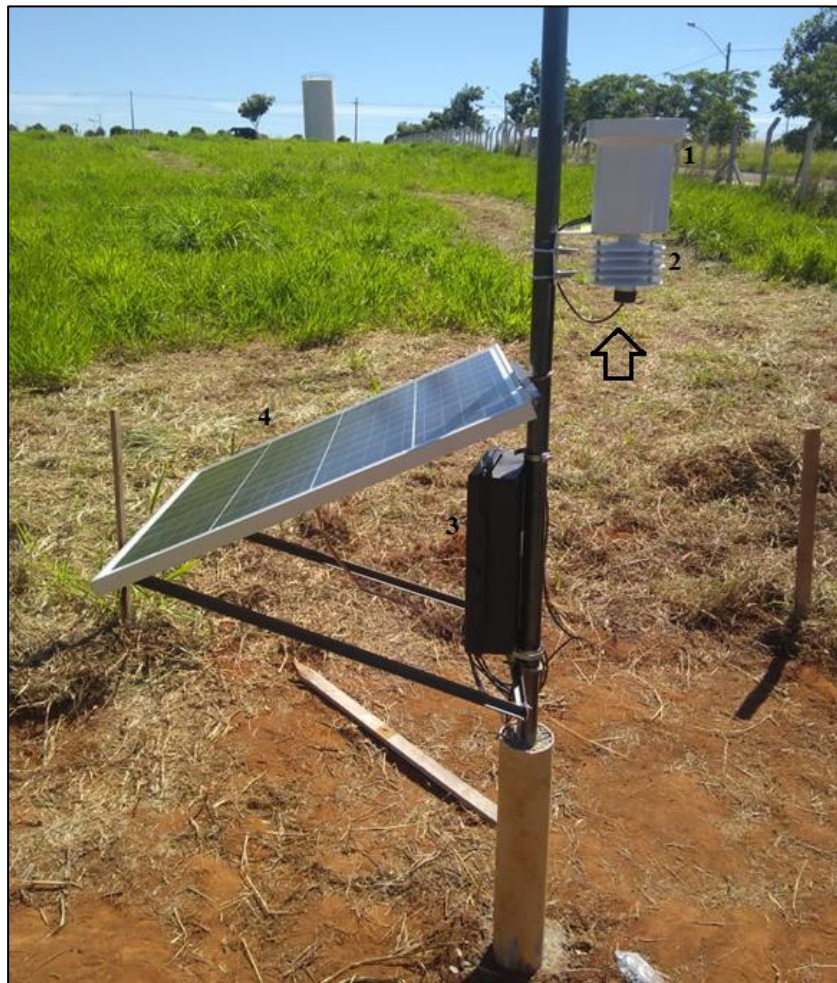
Figura 14 - Sensor instalado no Campus II
